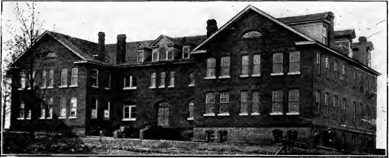
BALLARD INDUSTRIAL BUILDING—LIVINGSTONE COLLEGE
